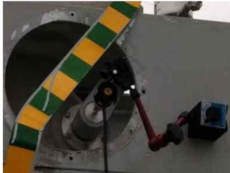
The arm of the SF6 circuit breaker has an angular displacement sensor connection port. Fix the U-shaped port in the screw hole correspondingly, and then fix the sensor with a universal joint. As shown below:
